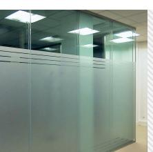
Virtually seamless joints between the glass panels with a transparent O-seam.
